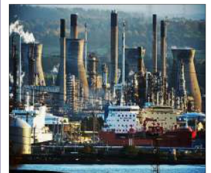
Refinery Petrochemical Plant
